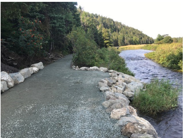
Trail Elevated to Prevent Flooding
